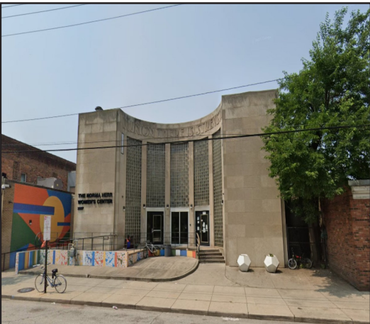
Cuyahoga County, the City of Cleveland, and Emerald Development and Economic Network, Inc. (EDEN) will join community partners to celebrate the grand opening of the newly renovated and expanded emergency shelter, the Norma Herr Center, 2219 Payne Avenue.
